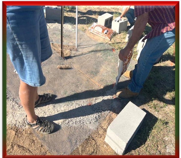
Lay crushed granite to level the cinder
