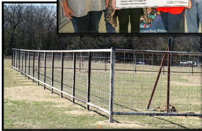
New Harvest Garden Fence Installed
