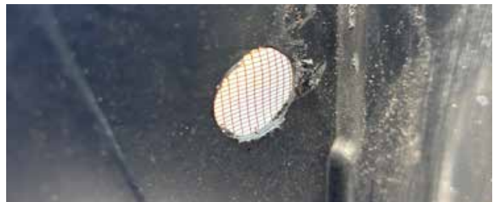
Close up view of screened ventilation holes MG Christie McGrath
