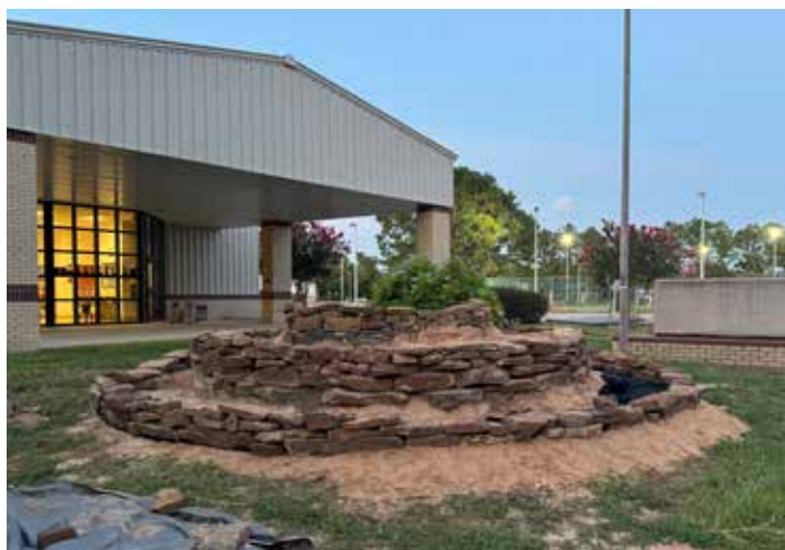
Lower tiers in progress MG Donna Merritt
