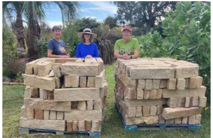
The edging stones were purchased and delivered. The outer edges of the beds were etched.
