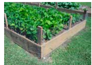
Box Out of 2x12 Lumber Supported at Corners by 4x4 Posts
