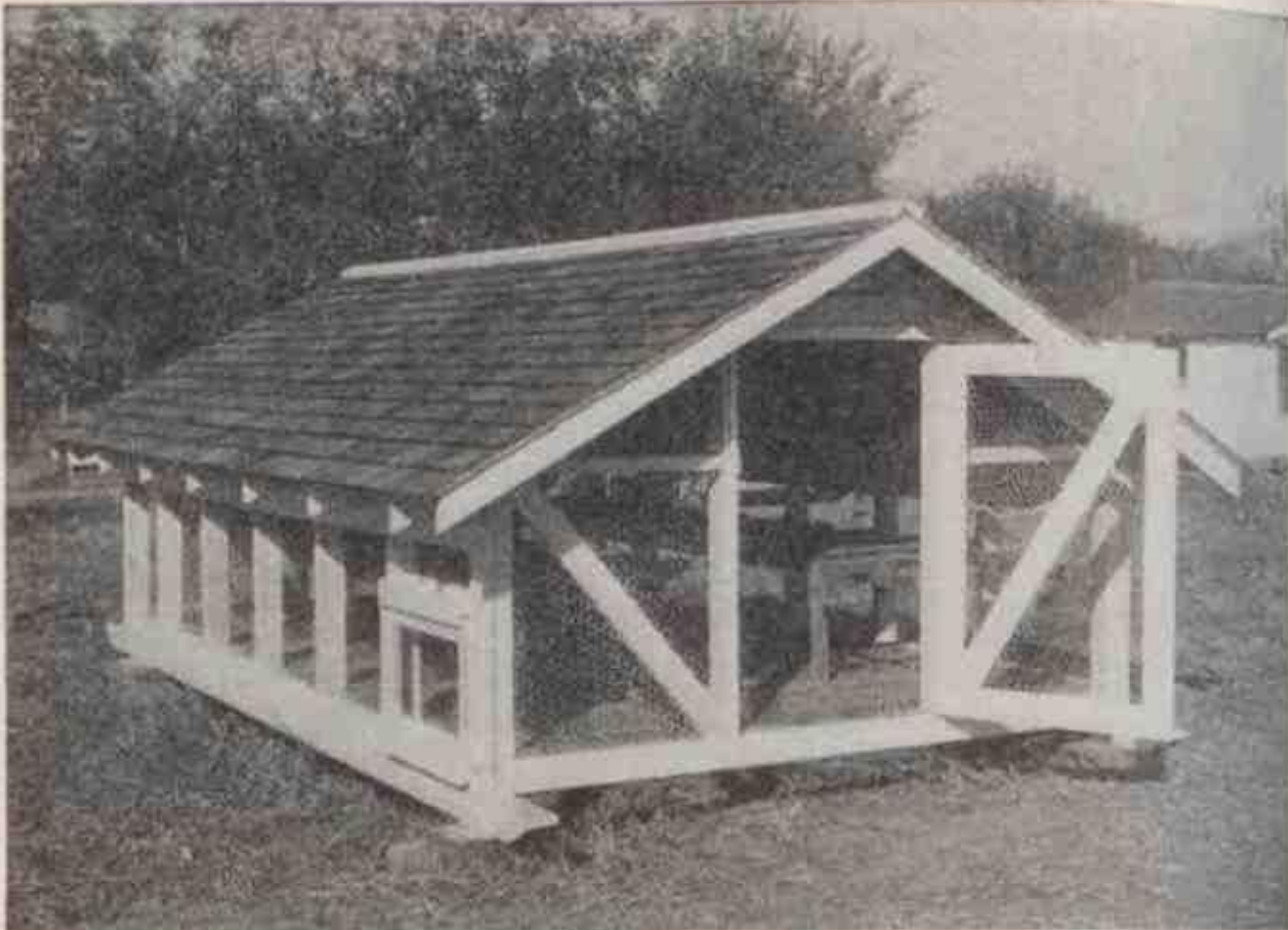
Fig. 104. A well-constructed range shelter built on skids to facilitate moving.
