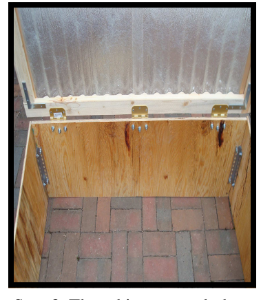
Step 3. Three hinges attach the lid to the cold frame box.
