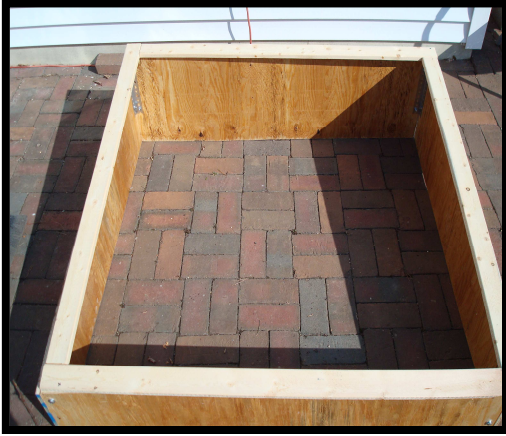
Step 1. Measure and cut lid frame boards to fit the top of the box. See Diagram A.
