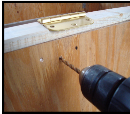
Step 3. Outside view. Pre-drill holes before attaching hinge to box and lid with dry wall screws.
