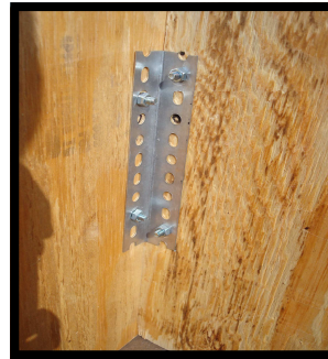
Step 2. Interior view of the angle steel attached to the box with four bolts.
