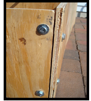
Step 2. Exterior view of the angle steel attached to the box. Use the flat-
