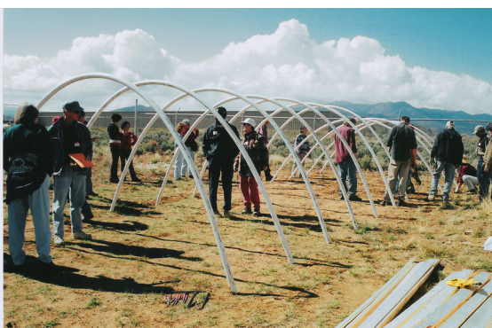
Figure 3. The hoop house structure takes shape.
