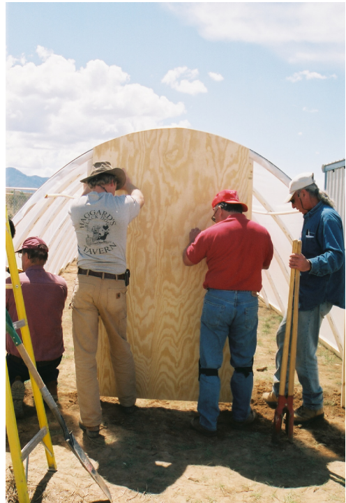
Figure 14. Attaching the front door to the hoop house.
