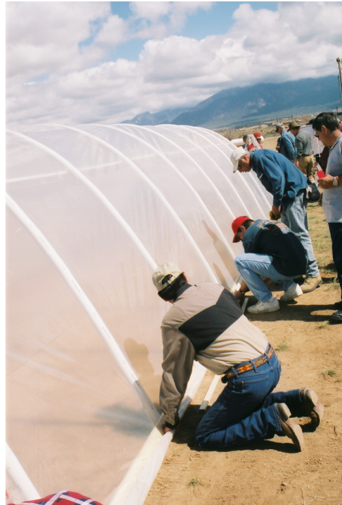
Figure 12. Attaching the plastic cover to the baseboards.
