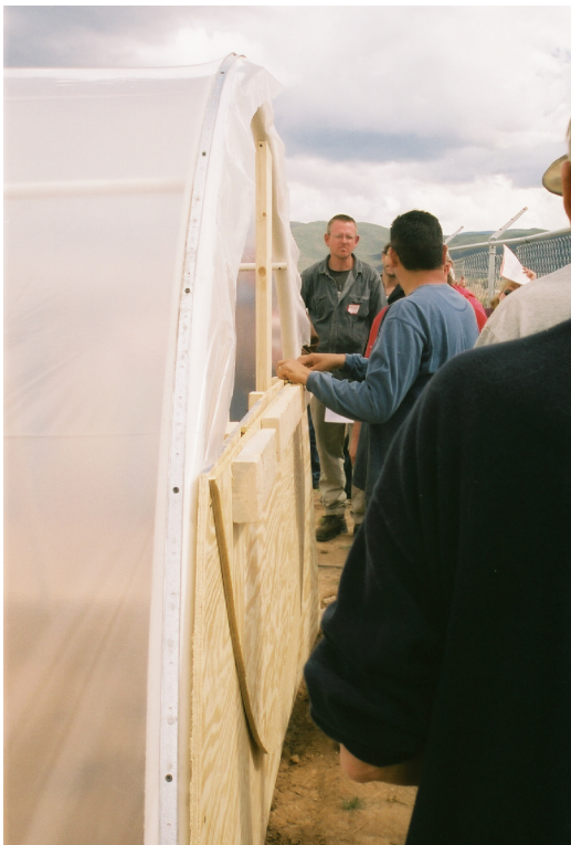
Figure 17. Window completed; hoop house completed.
