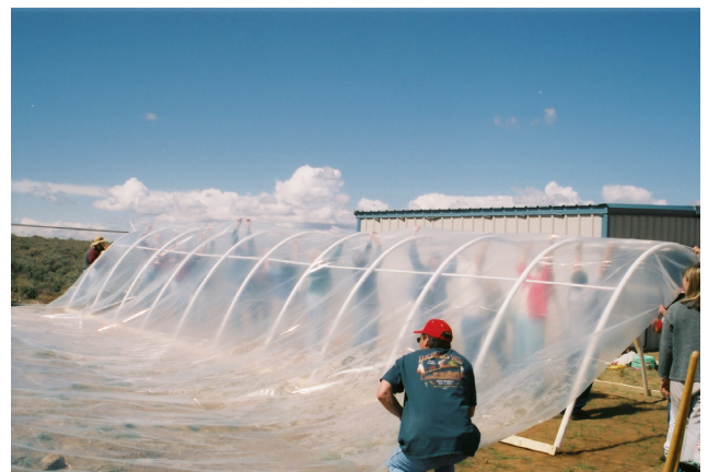
Figure 10. Covering the hoop house with 6-mil. plastic film.
