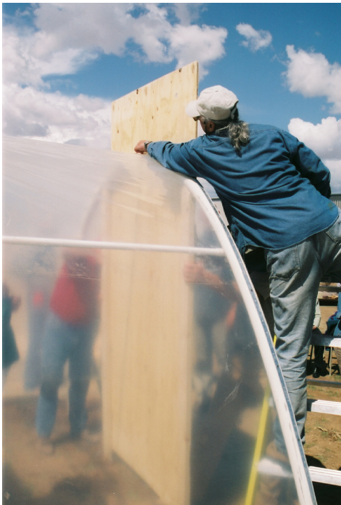
Figure 13. Marking the door to be cut.
