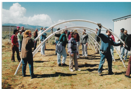
Figure 2. Bending the 2-in. x 20-ft. PVC pipe and setting them on 1/2-in. rebar stakes.
