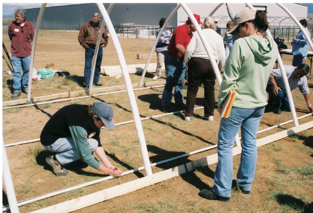
Figure 5. Laying out the tubular 3/4-in. braces.
