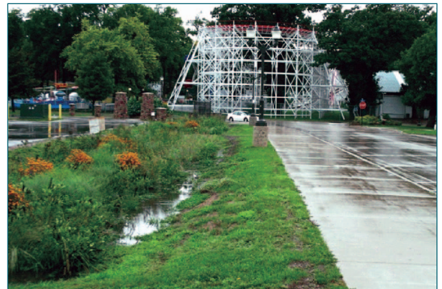
Figure 2. Rain garden built as an island in a parking lot. (Source: United States Department of Agriculture, Natural Resources Conservation Service)
