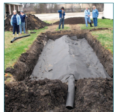
Figure 6. Placing the filter fabric.
