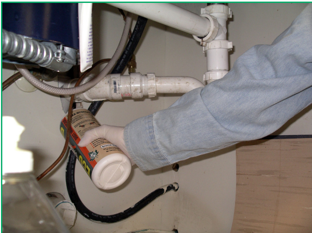
Figure 11. Applying dust to a wall void where plumbing pipes enter the wall.
