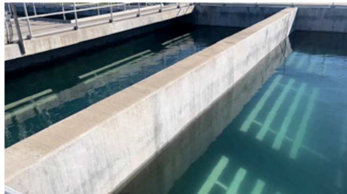
Figure 2 Floccing paddles helping separate particulate matter.
