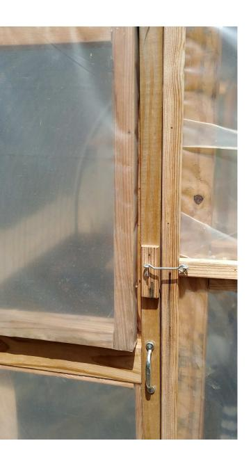
An inexpensive handle and a latch & screw-eye were the last things added to the doors.
