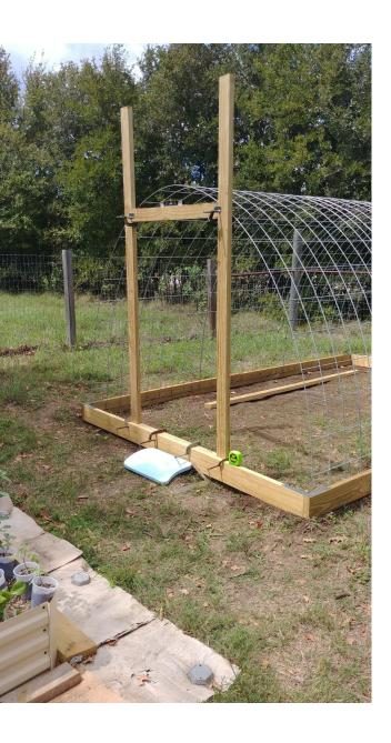
2x4s for the door have been clamped together, in order to mark for the angle cut needed at the top so the cattle panel can be stapled to the top of the door frame uprights.
