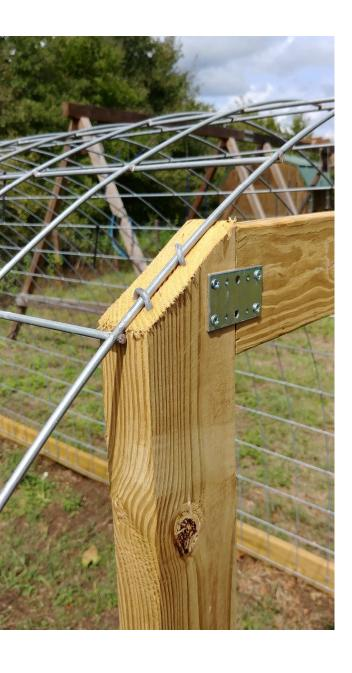
Door frame uprights cut to size and door frame top and bottom attached. Cattle panel stapled to door frame uprights.
