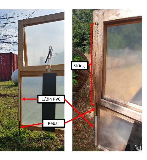
When it got warmer in the spring, I wanted to have the doors held open. A piece of 1/2in PCV attached to the inside of the door allows a piece of rebar to drop down to the ground to hold the door in place. A piece of string attached to the rebar holds it up when not needed.
