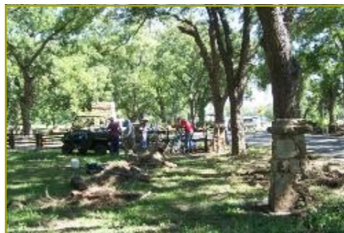
Fence tear down
